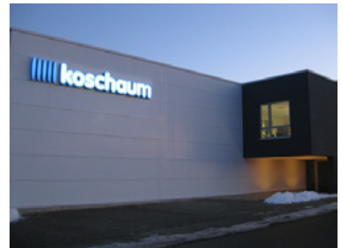
New administration building
