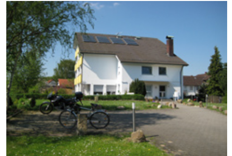
Officebuilding in Burgebrach
